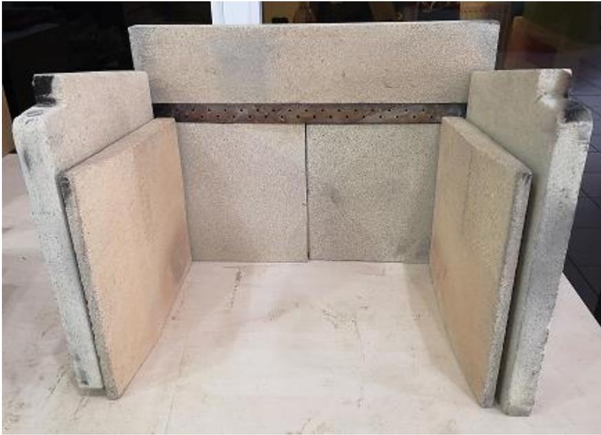
Figure 2 Baffle positioning
